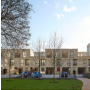
Alison Brooks Architects: Ely Court, London, UK Bild: Paul Riddle
